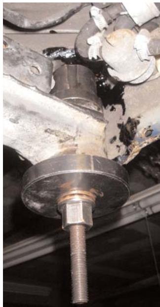
Photo #6 New bushing pressed into place.
